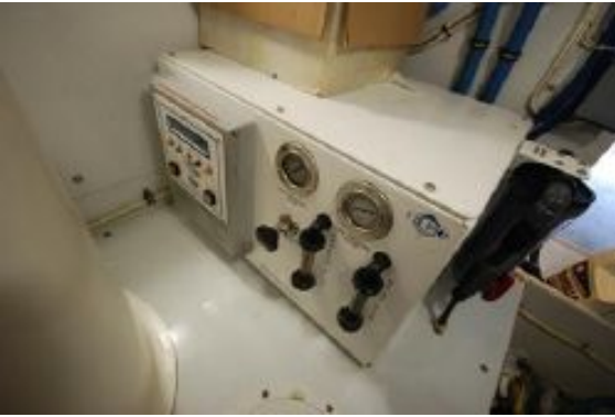
> Watermaker/ Pump Room
