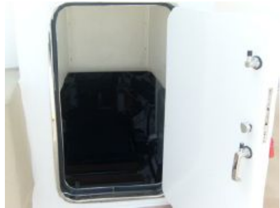
> Engine room access
