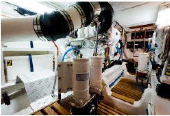
ENGINE ROOM VIEW 1
