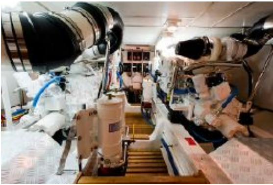
ENGINE ROOM VIEW 3
